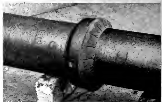
A Neat and Impervious Joint
